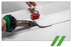
directly to the sheet metal by welding. Where the sheets are butted together, they are connected with strips of KÖSTER TPO U at least 10 cm wide. This is completely welded.
