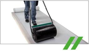
// The Membrane is then be pressed on over the entire surface, ideally with a pressure roller.
